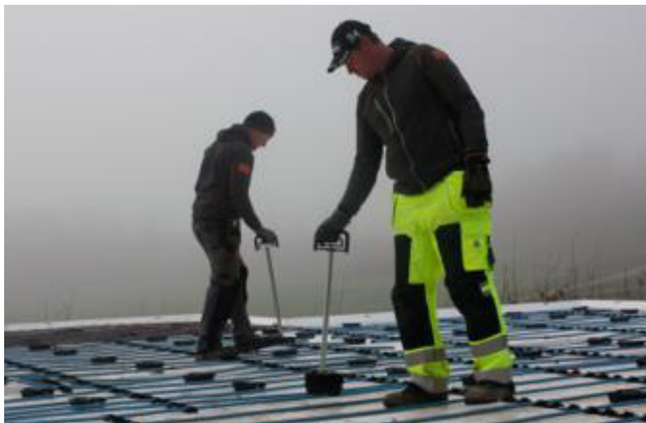
With a Speedies Dropstick, ergonomics are improved and working time is reduced by 75%
